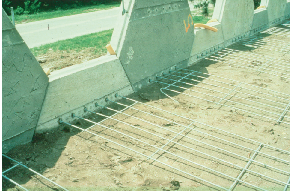
Figure 10.1.9 Mechanically Stabilized Earth Wall Under Construction
