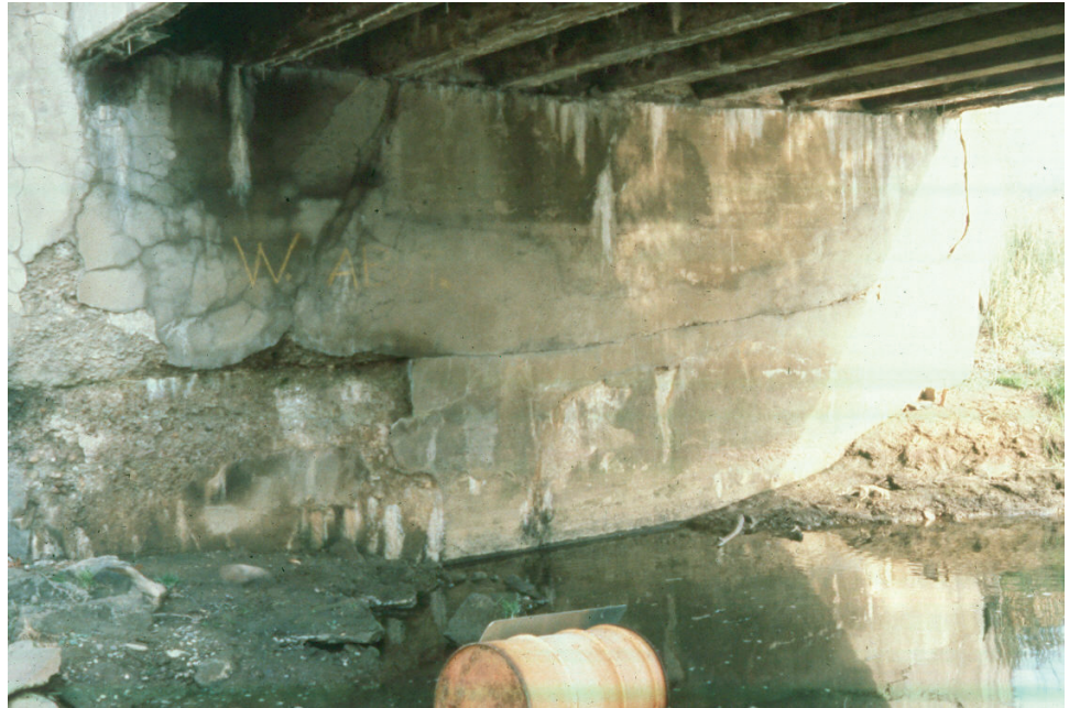
Figure 10.1.12 Plain Unreinforced Concrete Gravity Abutment
