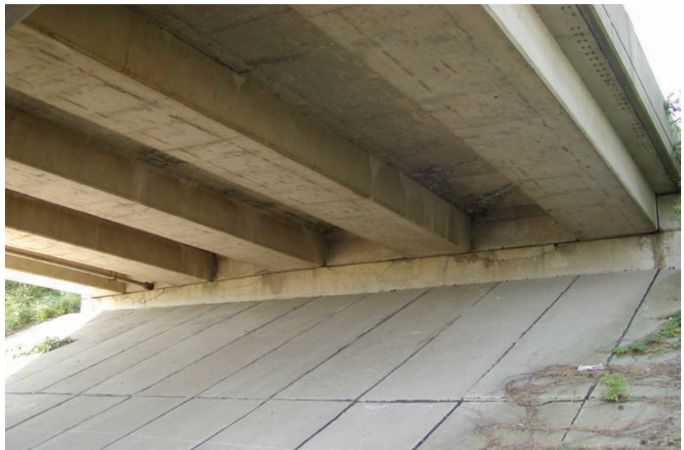
Figure 10.1.4 Stub Abutment
