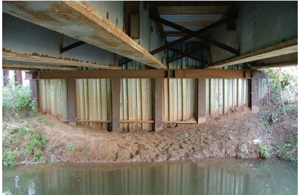
Figure 10.1.16 Steel Abutment
