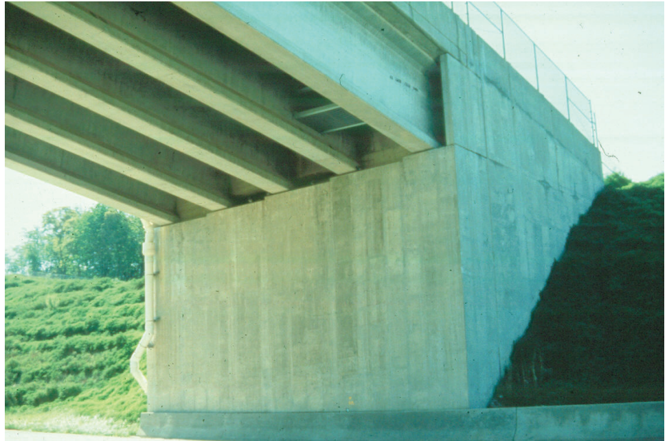
Figure 10.1.3 Full Height Abutment
