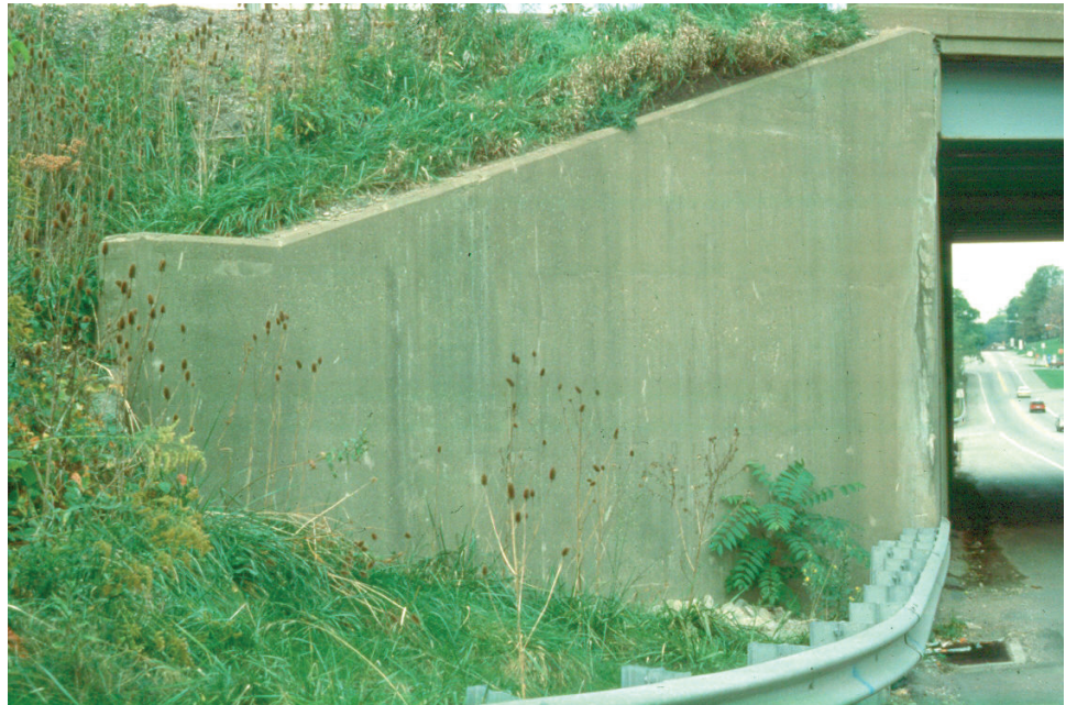
Figure 10.1.41 Typical Wingwall
