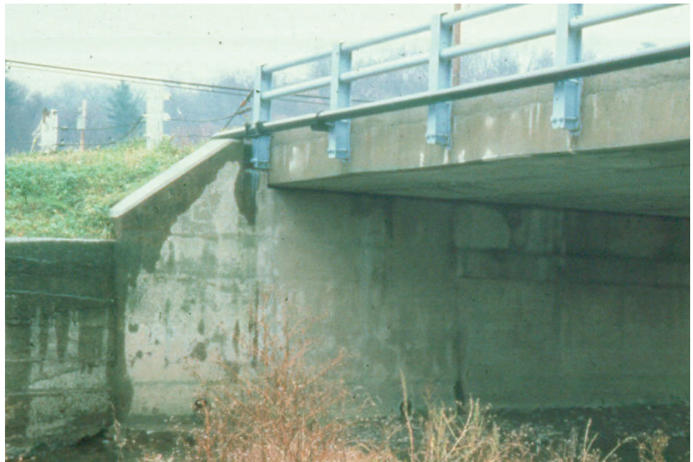
Figure 10.1.45 Integral Wingwall
