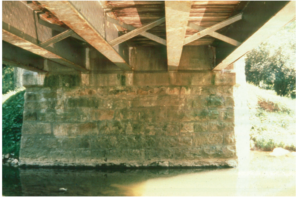
Figure 10.1.14 Stone Masonry Gravity Abutment
