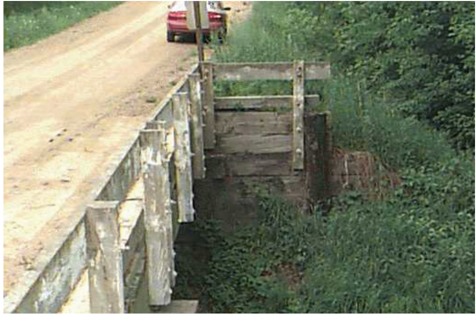
Figure 10.1.55 Timber Wingwall
