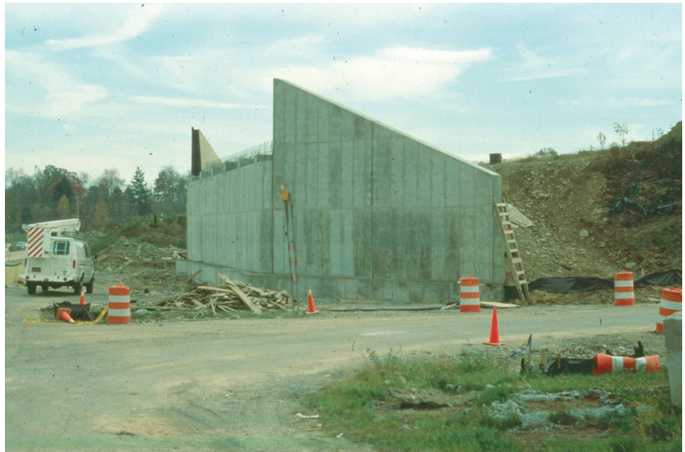
Figure 10.1.13 Reinforced Concrete Cantilever Abutment
