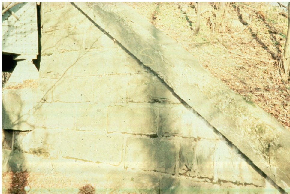
Figure 10.1.47 Masonry Wingwall
