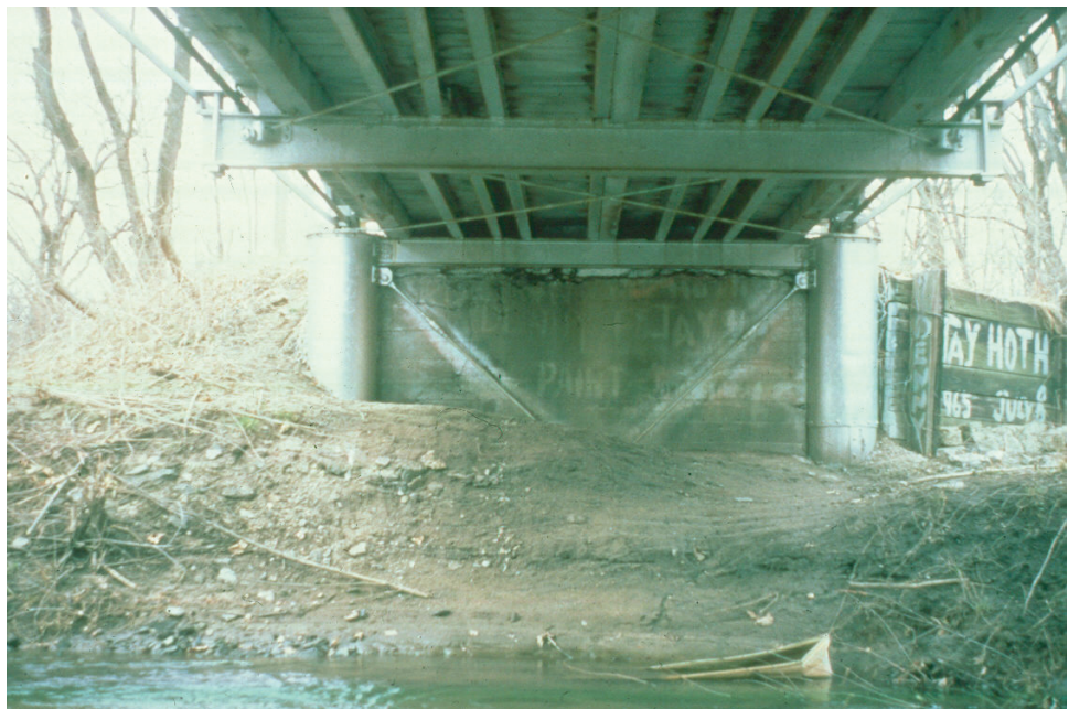
Figure 10.1.35 Steel Abutment
