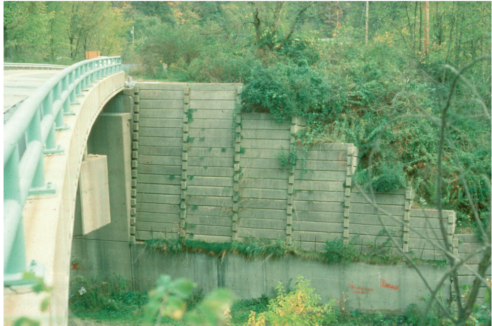
Figure 10.1.42 Straight Wingwall
