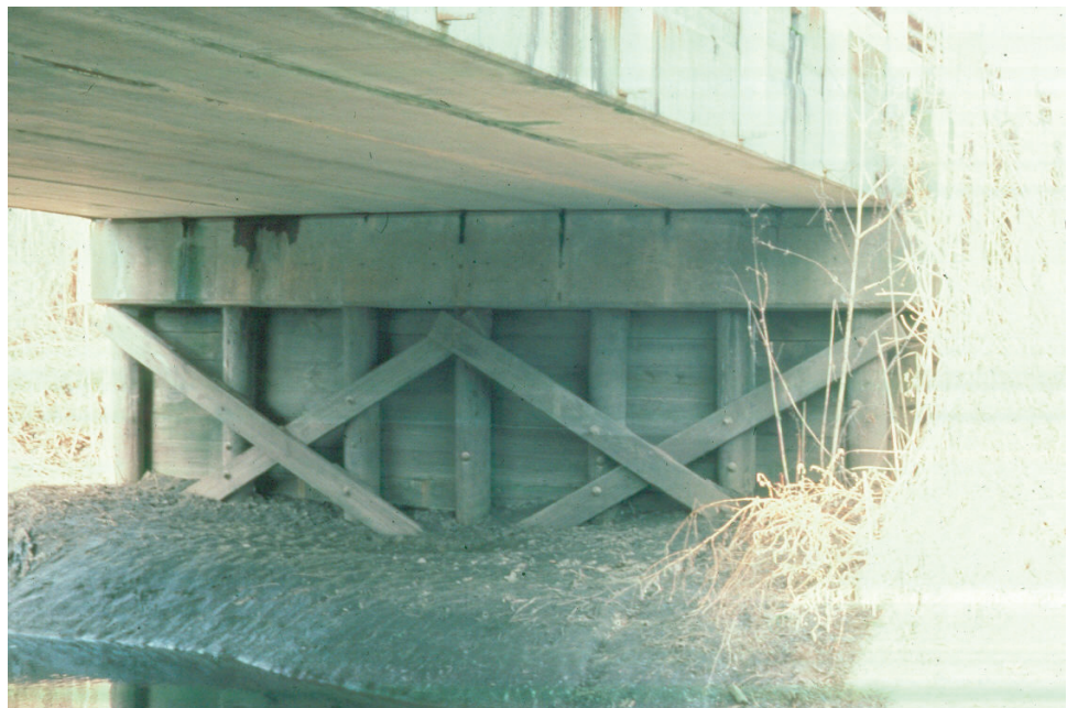
Figure 10.1.15 Combination: Timber Pile Bent Abutment with Reinforced Concrete Cap
