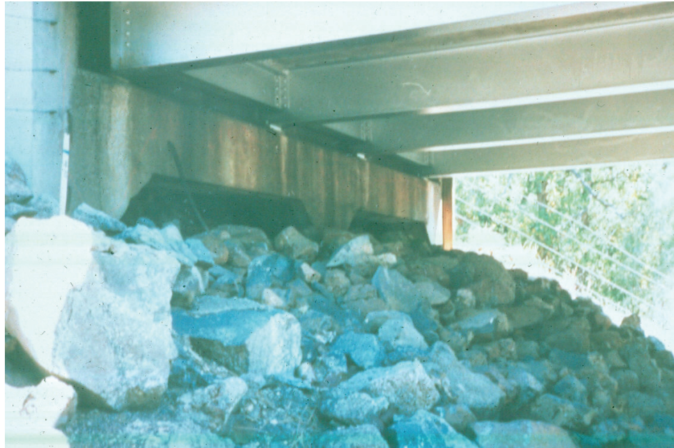
Figure 10.1.5 Open Abutment
