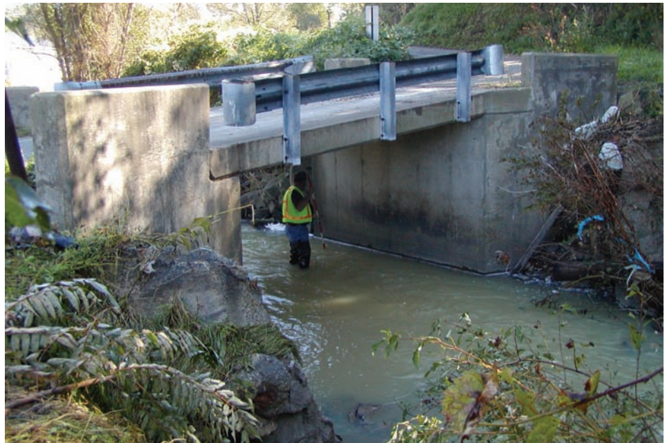
Figure 10.1.40 Inspector Checking for Scour
