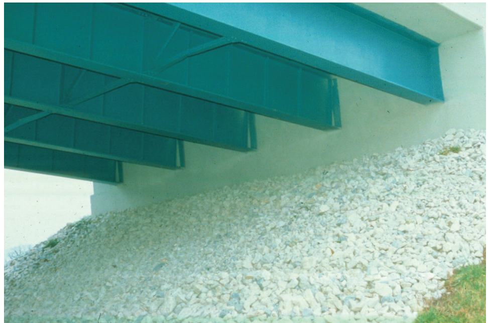
Figure 10.1.7 Integral Abutment
