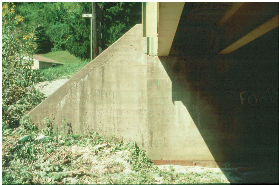
Figure 10.1.43 Flared Wingwall
