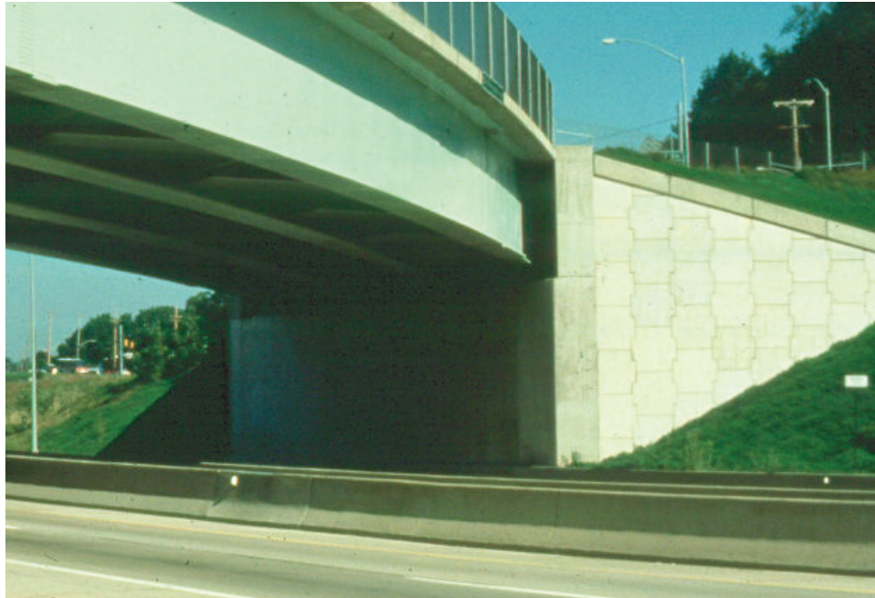
Figure 10.1.46 Independent MSE Wingwall
