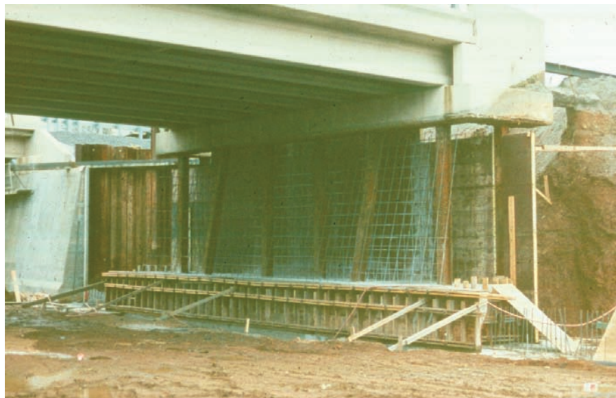
Figure 10.1.21 Stub Abutment on Piles with Piles Exposed
